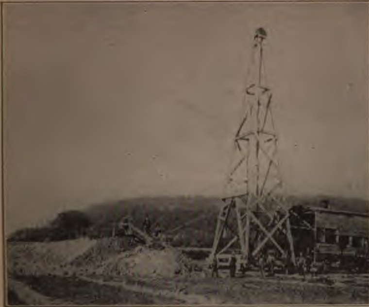
Tower Excavator. Figure 67.
